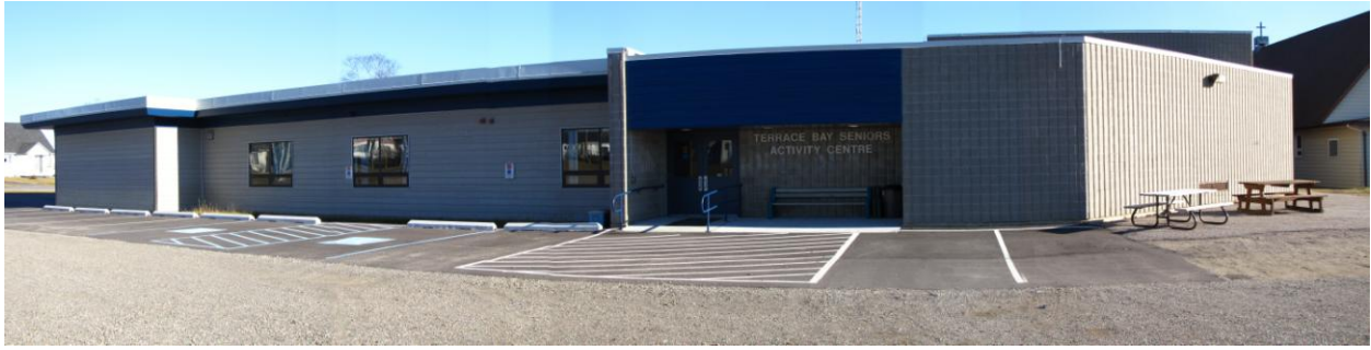
Rear Entrance (Handicap Accessible)
