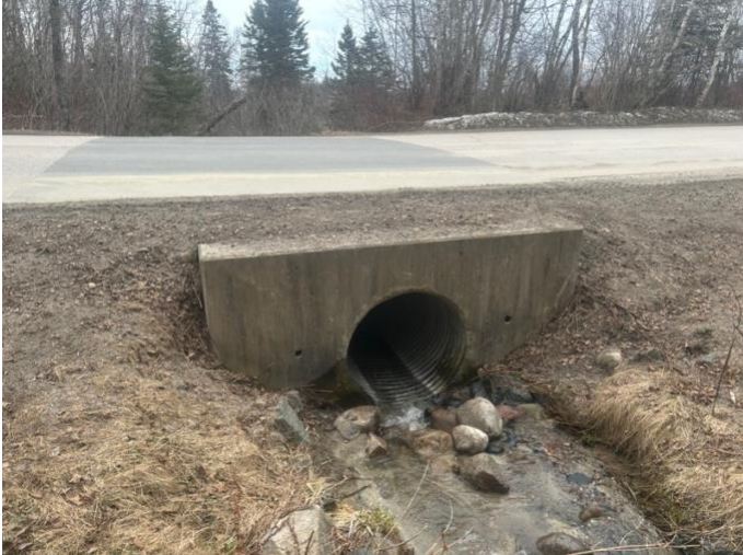
Figure 13: Beach Road Culvert
