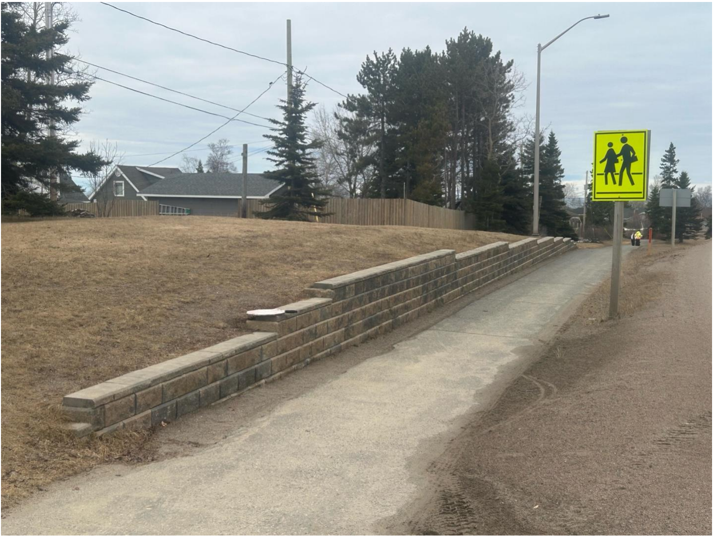
Figure 14: Retaining wall adjacent to multi-use path
